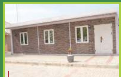
RISE Project office (Portacabin) constructed within TACA premises
